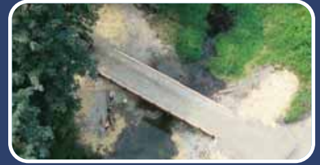
A bird's-eye view of the new 2024 bridge on Lower Day Slough.
