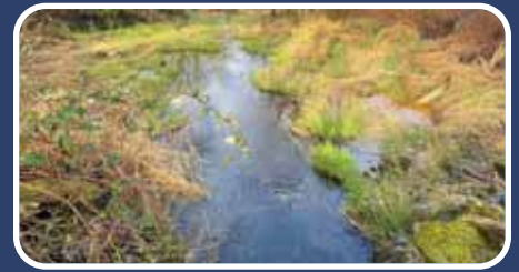
Looking downstream at Lower Day Slough from the culvert that was replaced with a bridge in July of 2024.
