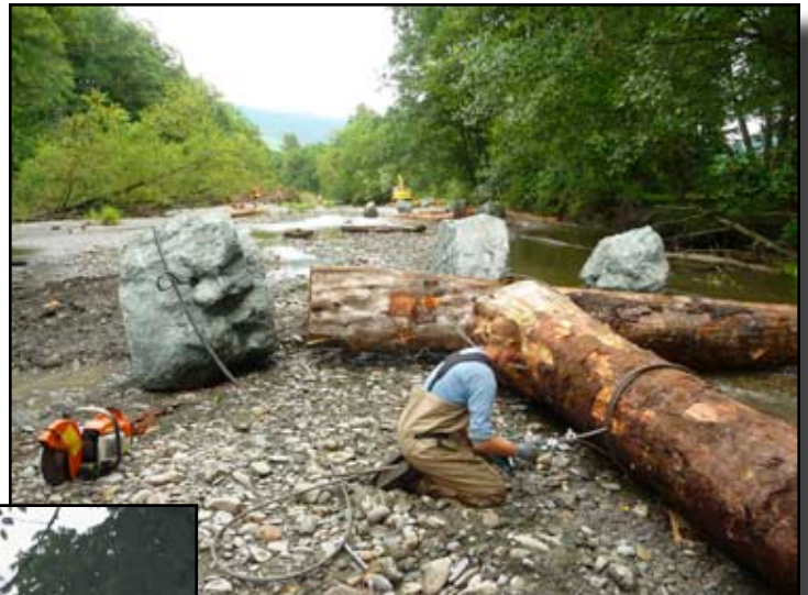
Cabling logs together
